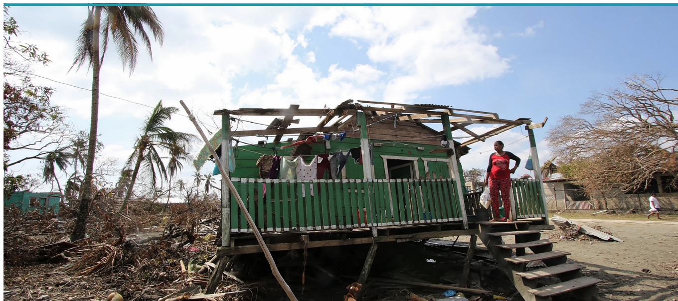
Destruction caused by Hurricane Eta in Nicaragua in November 2020. EMPOWER supported Caritas Nicaragua in a rapid emergency shelter and WASH response to the Category 4 hurricane. Photo by Katlyn Holland/CRS
